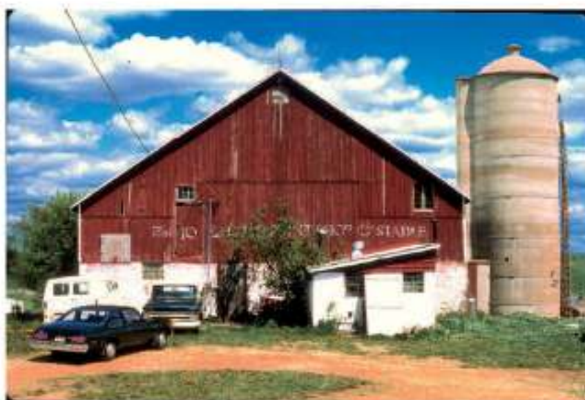
Jones Road Printshop and Stable near Barneveld, WI (1971 - 1984) photo credit Jim Perotto
